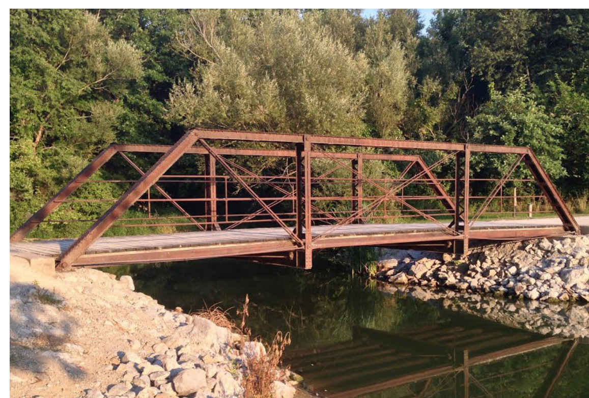
Pony Truss Bridge
