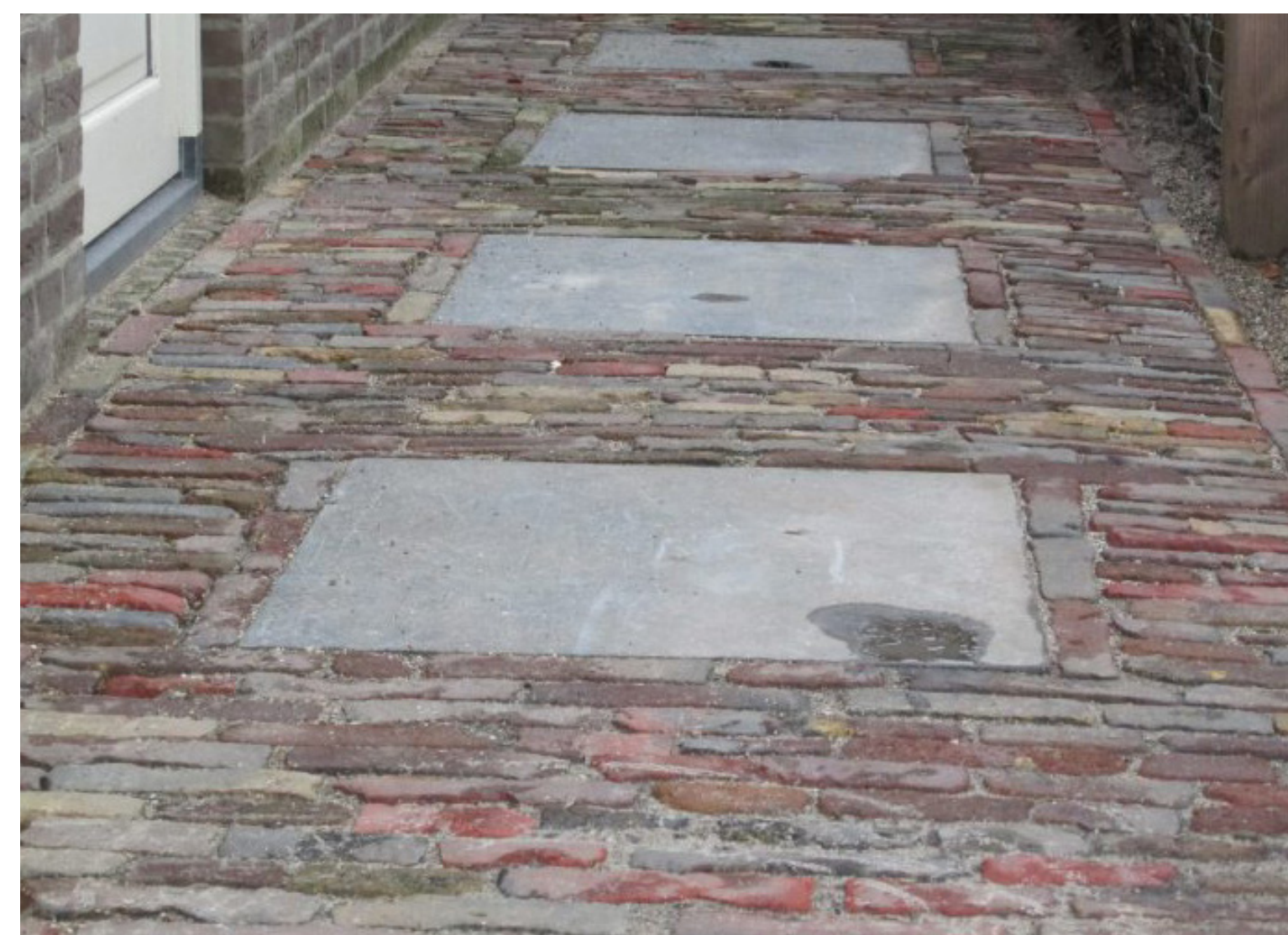
Brick with Concrete Accents
