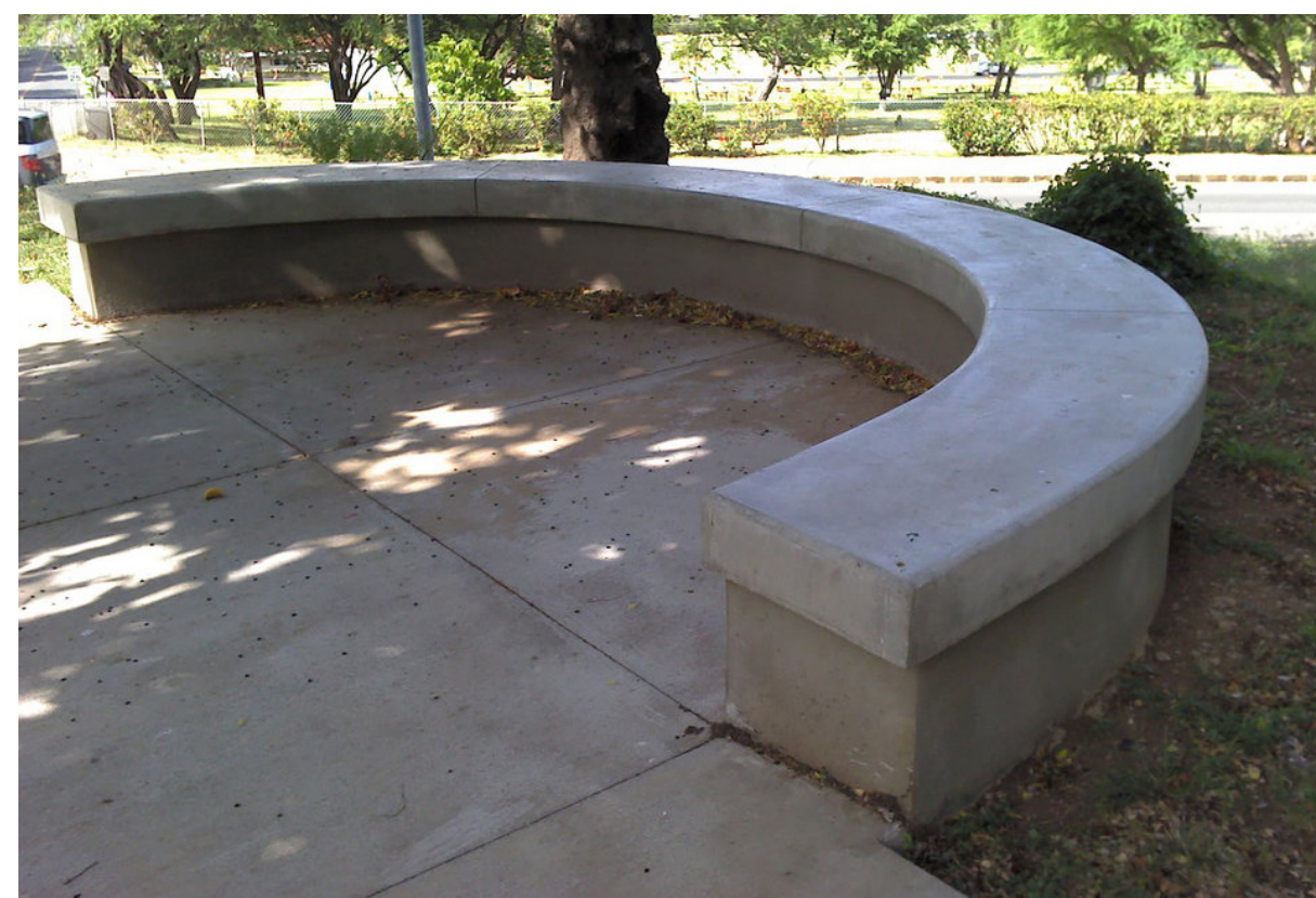
Precast Concrete Seat Wall
