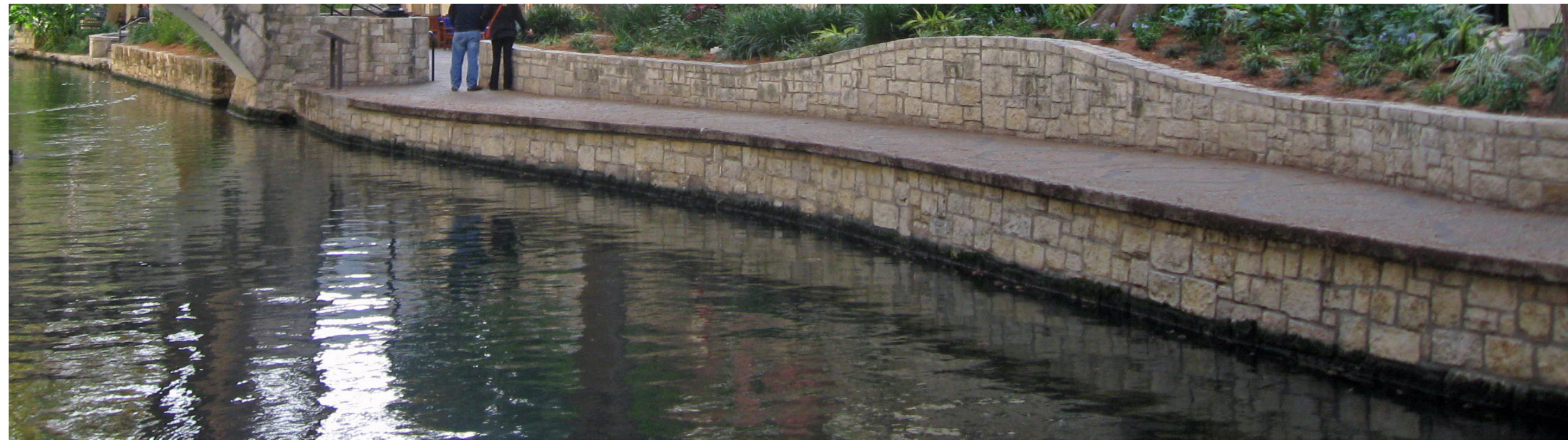
Limestone Wall with Concrete Walk
