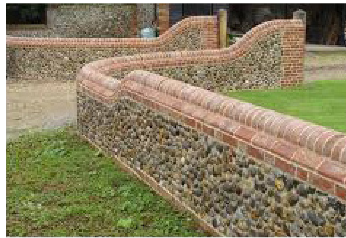
Cobble Stone wall with Brick Coping
