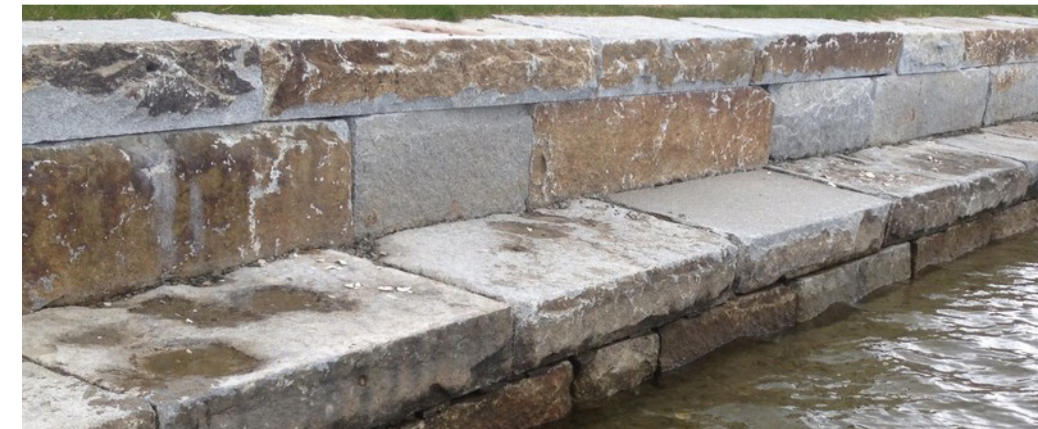
Rough Stone Block Wall / Coping
