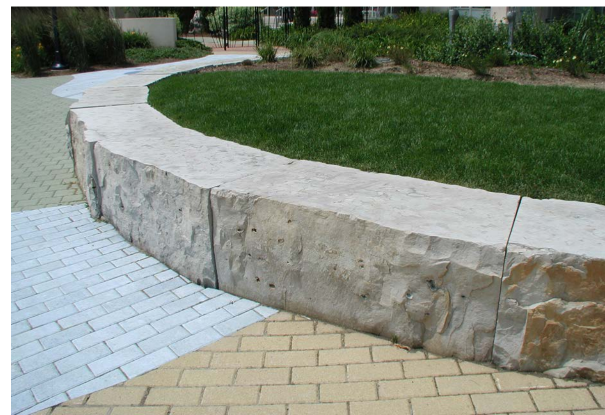
Limestone Block Wall
