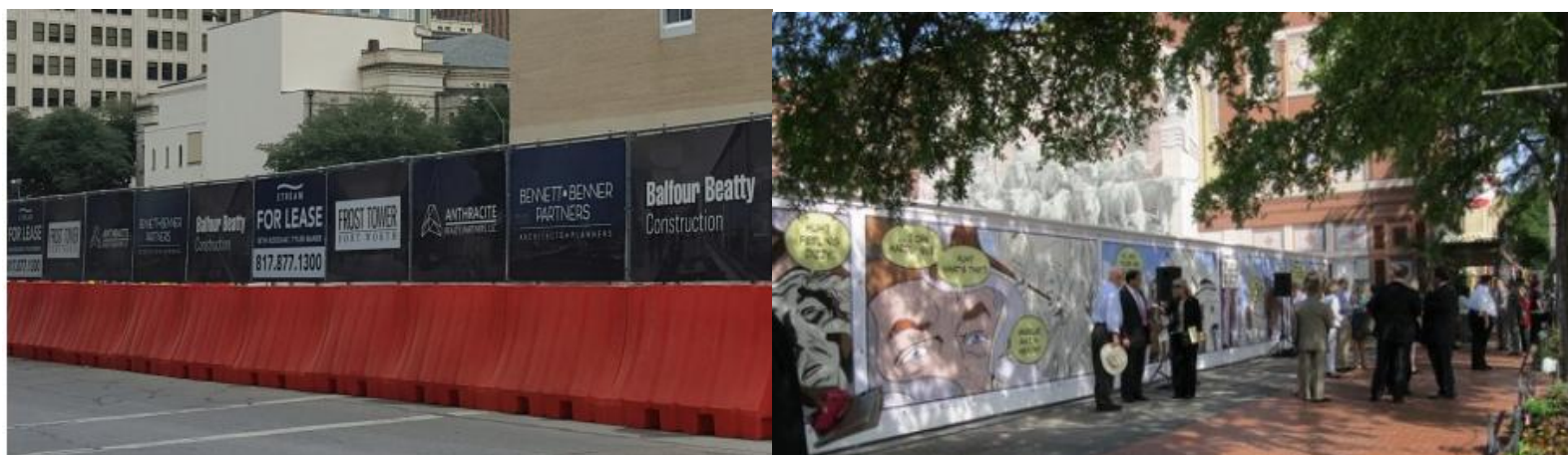
Fig. 10-10: Examples of acceptable construction site screening.
