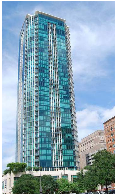
THE TOWER CONDOS - 488'
